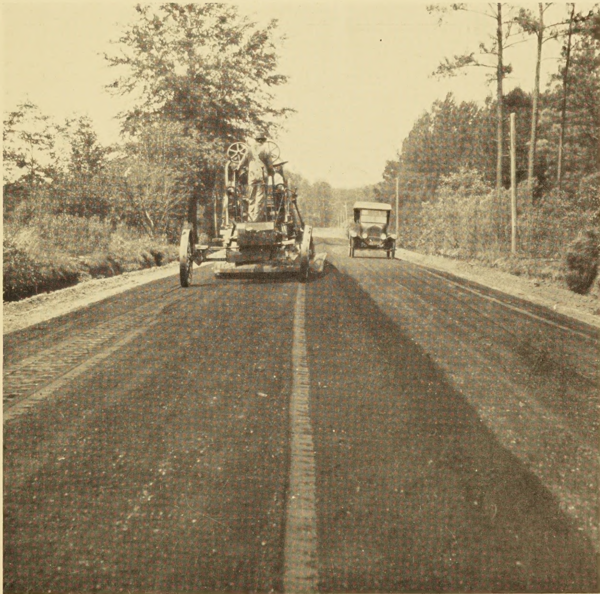
MIXING OPERATIONS ON A BITUMINIOUS EXPERIMENTAL ROAD IN SOUTH CAROLINA
